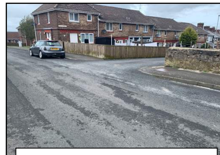
Site Photo – taken Victoria Road April 2024
